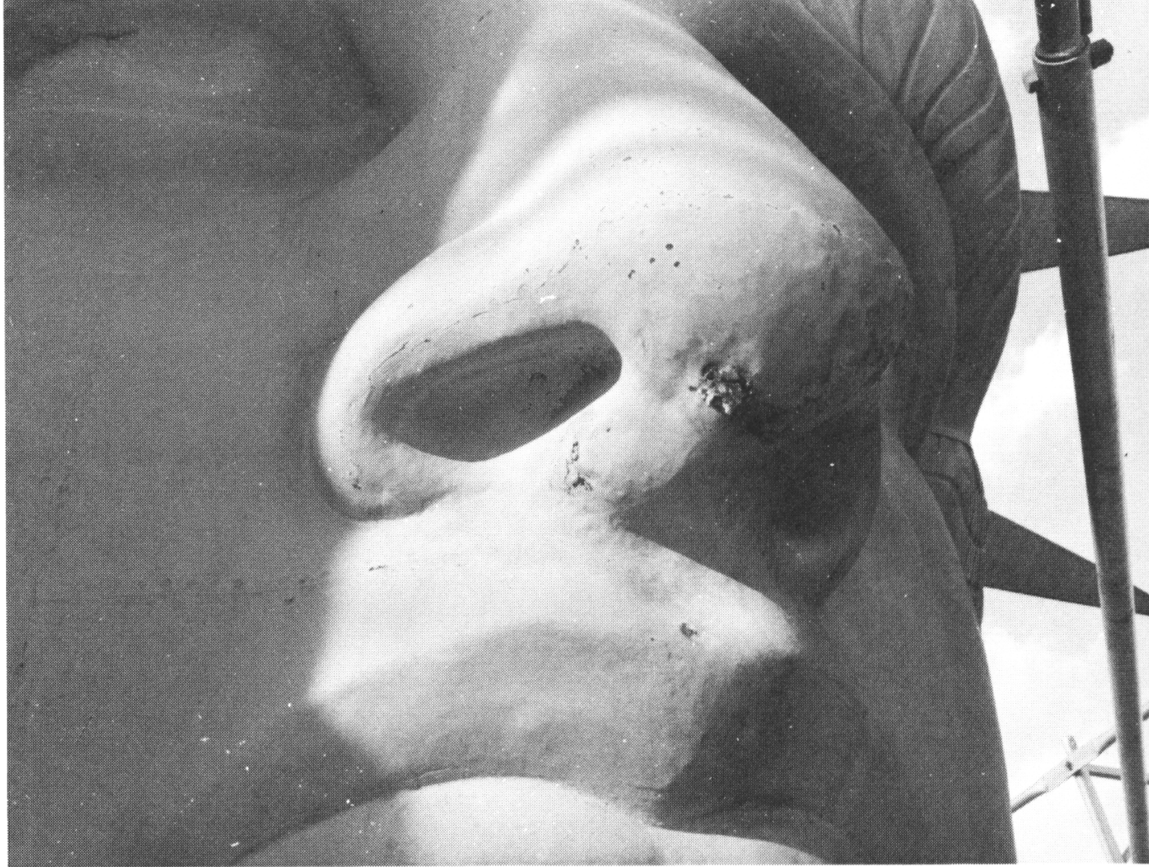
Moisture that collected on the inside of the Statue of Liberty caused galvanic corrosion of armature in contact with the copper skin. The copper skin on the nose was ruptured due to mechanical forces of the resulting corrosion products.
